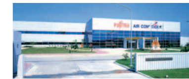
Fujitsu General (Thailand) Co., Ltd. Fujitsu General Engineering (Thailand) Co., Ltd.
